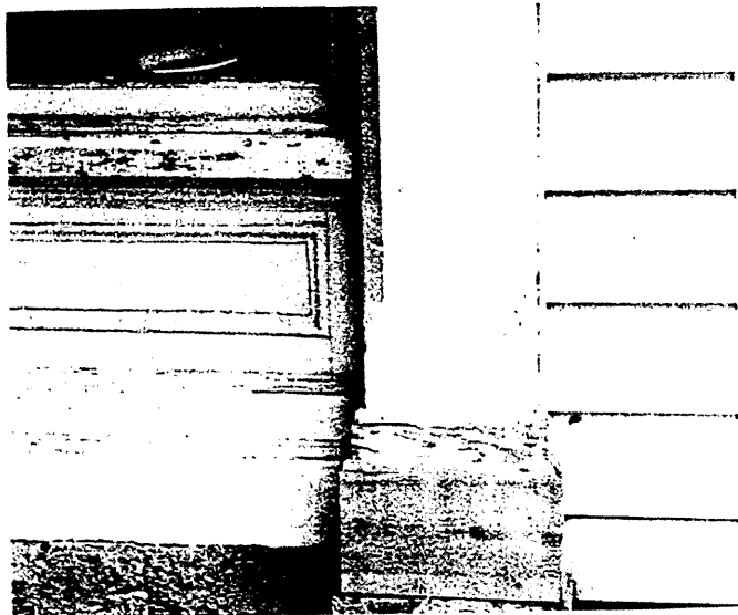
Figure 9. Rather than replace an entire wooden storefront when there is only localized deterioration, a new wooden component can be pieced-in, as seen here in this column base. The new wood will need to be given primer and top coats of a high quality exterior paint—either an oil-base or latex system. Also wood that is flaking and peeling should be scraped and hand-sanded prior to repainting. Photo: H. Ward Jandl
