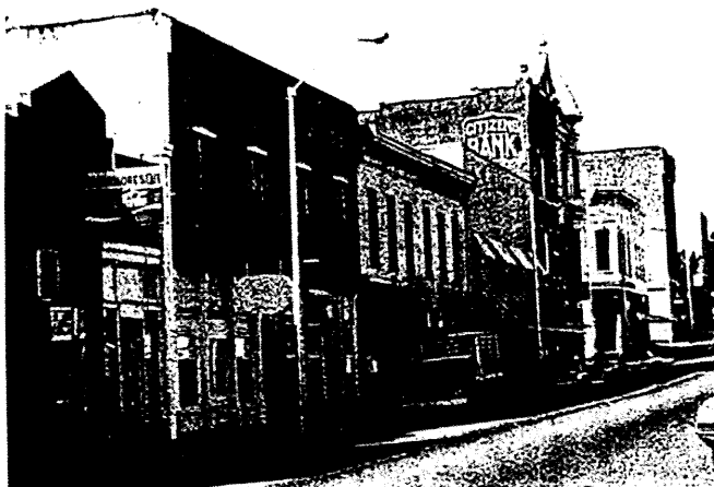
Figure 1. Inappropriate storefront alterations over the years—metal cladding, oversized signs and canopies—have detracted from the character of this historic district in Van Buren, Arkansas. A carefully considered rehabilitation plan for Main Street, including the removal of poorly designed signs, false fronts and the selection of an appropriate exterior paint color palette, serves to enhance the visual environment and preserves the district's sense of time and place. Photo above: Bob Dunn; Drawing, David Fitts
